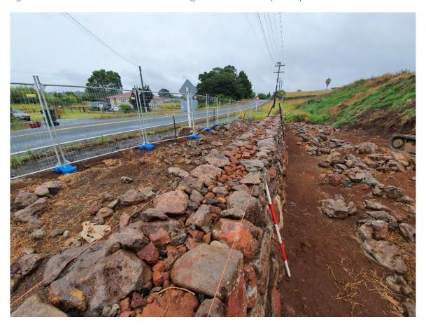
Figure 36: Reconstruction of stone wall.
