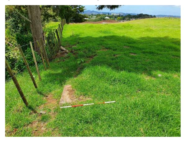
Figure 57: Concrete slabs and blocks pushed into small swale.
