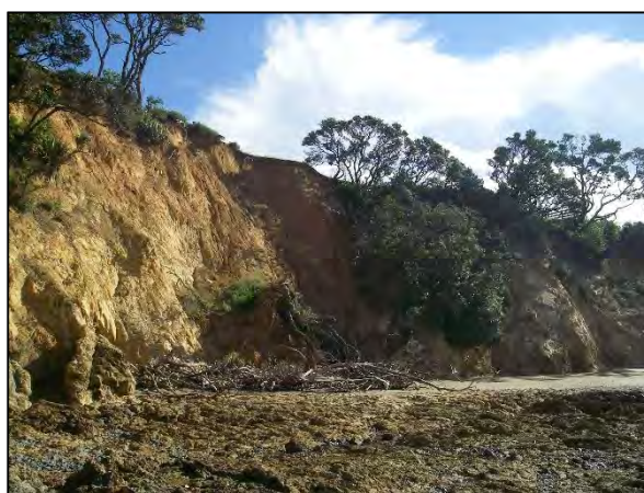
Site Photograph C (south cliff shoreline)
