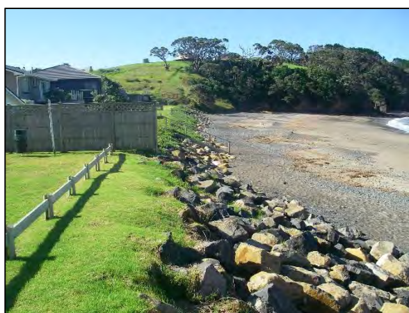
Site Photograph B (centre)
