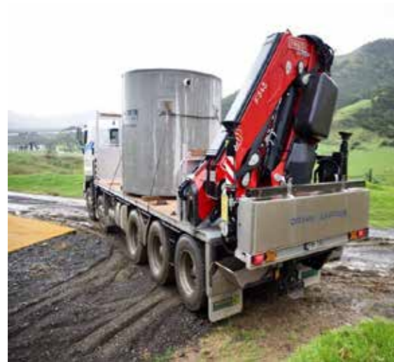
The tank is swung into place in its new position above the yellow grated platform of the vehicle hygiene station.
