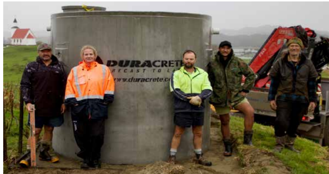
The tank install crew with Pawarenga church in the background.
