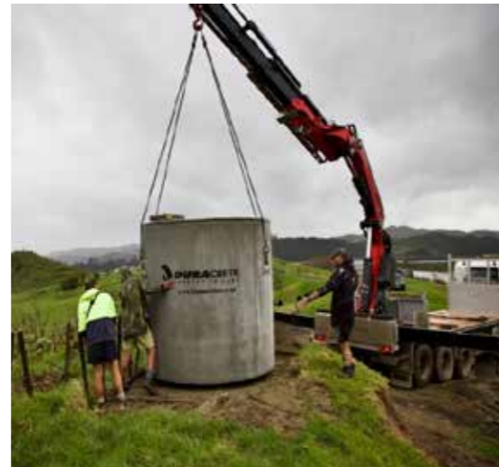
The tank is swung into place in its new position above the yellow grated platform of the vehicle hygiene station.
