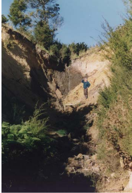
Gully erosion near Otaika
