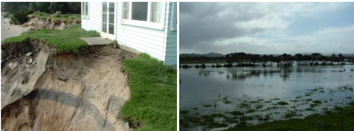
Erosion threatening dwelling at Omapere Beach following the storm event (left) and coastal inundation of land bordering the Hokianga Harbour (right).
