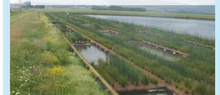
New floating wetlands installed on the Kaitiāia sewage pond to reduce blue-green algae.
