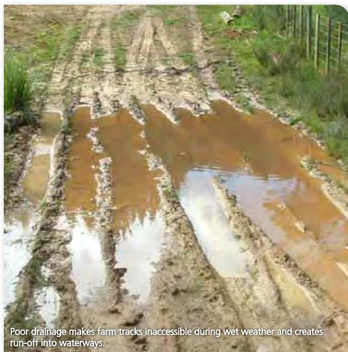
Poor drainage makes farm tracks inaccessible during wet weather and creates run-off into waterways.
