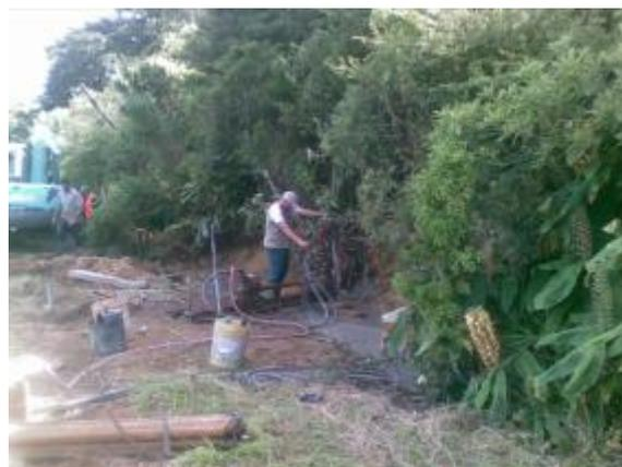
**A drill crew installing horizontal drainage to reduce soil saturation and help mitigate instability at the Bells Hill slip, Kaitiāia**
