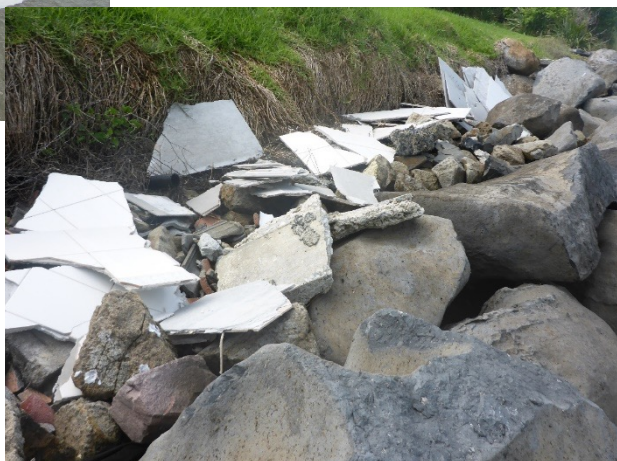
Council responded to 46 complaints of unauthorised structures in the coastal marine area between 2019 and 2023, including this unauthorised seawall, constructed using building debris as backfill.
