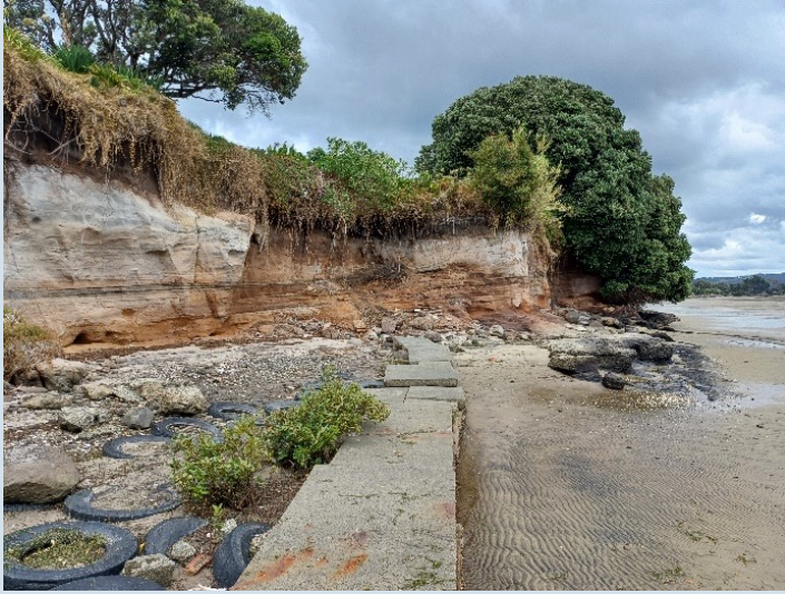
An unauthorised sea wall at One Tree Point, comprising, concrete blocks, tyres and material containing asbestos.
