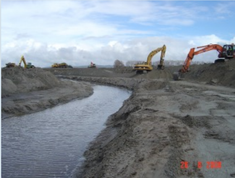
In 2008 a new inland marina was constructed at Marsden Bay, by excavating large canals on agricultural land and then flooding them with saltwater.
