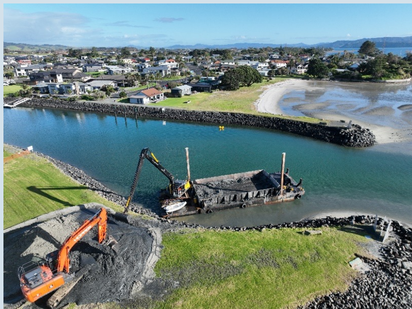
Ongoing maintenance dredging is required to maintain access to the marina via a human-made channel across Marsden Bay.
