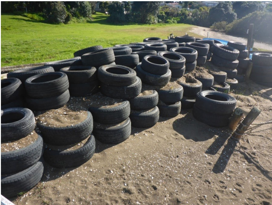
An unauthorised Seawall at Tinopai constructed out of old vehicle tyres was removed following enforcement action by Council.
