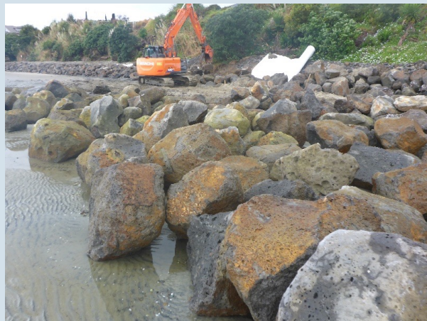
Whangārei District Council spent more than half a million dollars to replace an old timber wall at One Tree Point with a rock revetment in 2017 30 .
