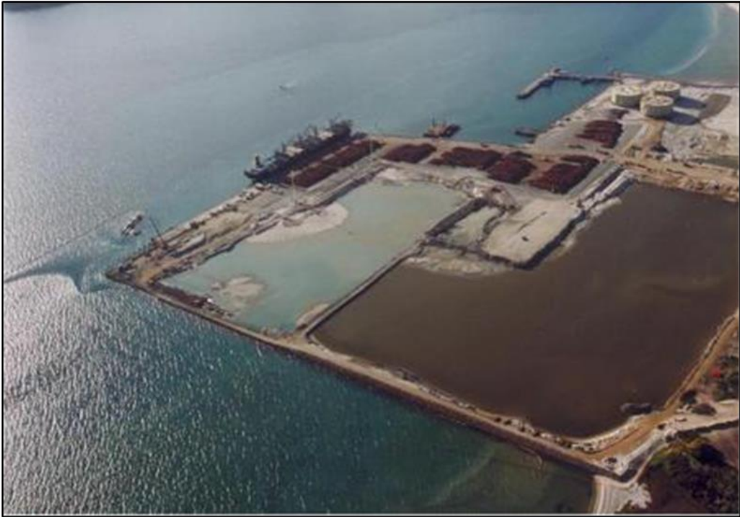
Figure 10: Sand being discharged using the perimeter bund method (with several internal paddocks) during original reclamation works at Northport
