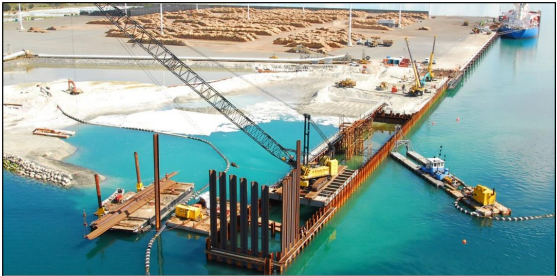
Figure 5: Berth 3 under construction showing the two parallel steel walls prior to backfilling
