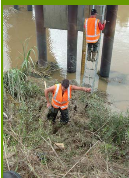
Regional Council staff installing a water level recorder.
