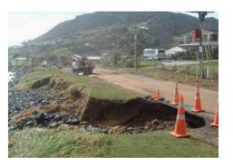
Substantial erosion also affected the Omapere foreshore, with differential erosion of between 1 - 4 metres on average along most of the Omapere foreshore. At least one dwelling was put at direct risk from this event with the concrete foundation overhanging the edge of the eroded dune scarp, as shown in the photograph below.
