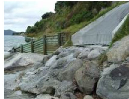
Seawall and stormwater outflow at One Tree Point.
