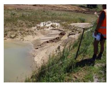
Photo: Poorly maintained sediment pond - minor non-compliance
