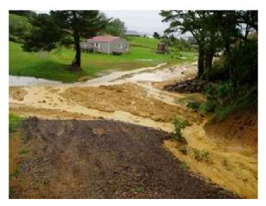
Photo: Sediment run-off from earthworks activity with no sediment control features - significant non-compliance
