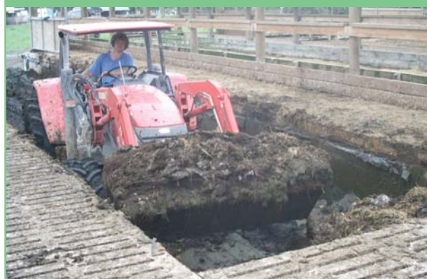
REMOVING DRIED EFFLUENT FROM BUNKERS UNDER CONCRETE SLATS OF HERD HOME
