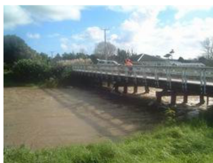
Whangatane Spillway in flood
