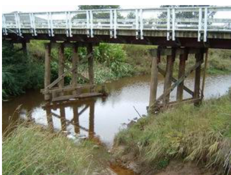
Whangatane Spillway before flood
