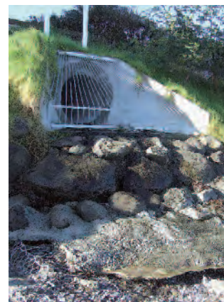
Stormwater drains deliver potential contaminants to the sea.
