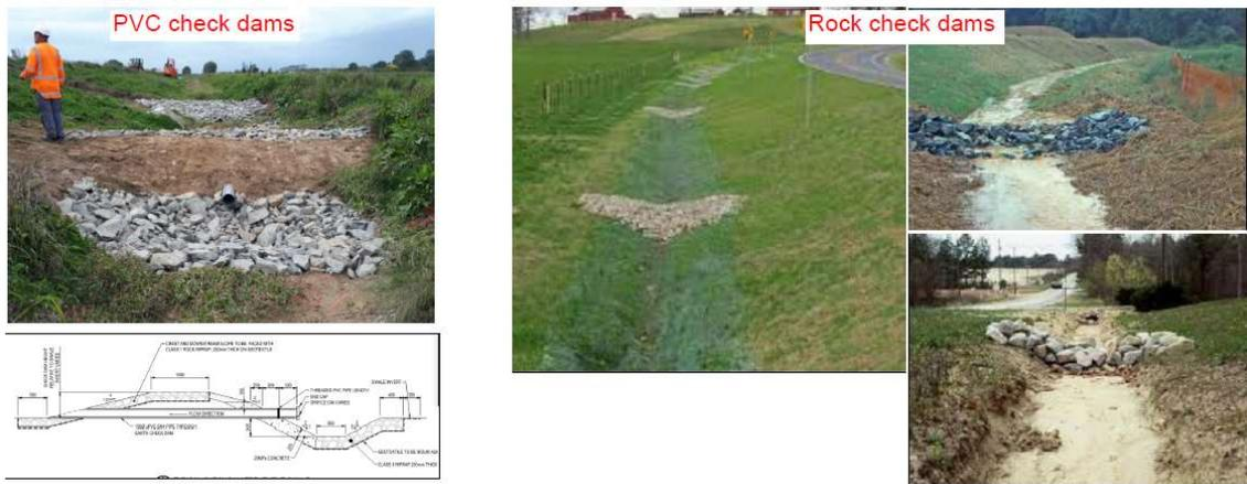
Figure 2: Examples of check dams constructed in swale drains to retain water. Images supplied by Beca.
