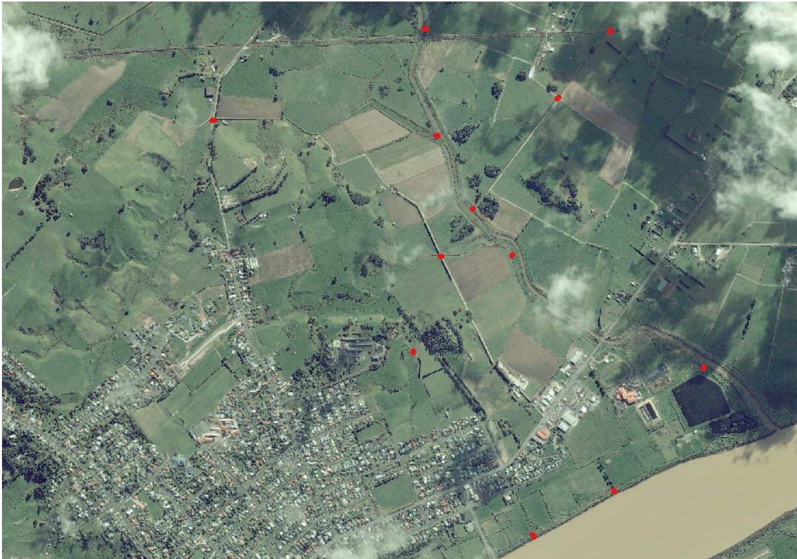
Figure 17: Positions of culverts surveyed on the Awakino floodplain in 2015 and included in the model
