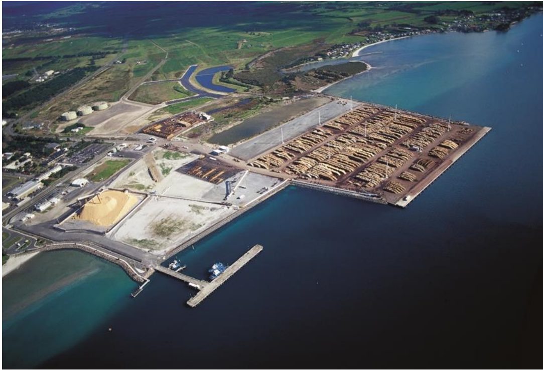
Figure 9: Aerial photograph showing Berths 1 & 2
