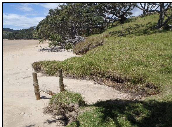
Site Photograph C (western end)
