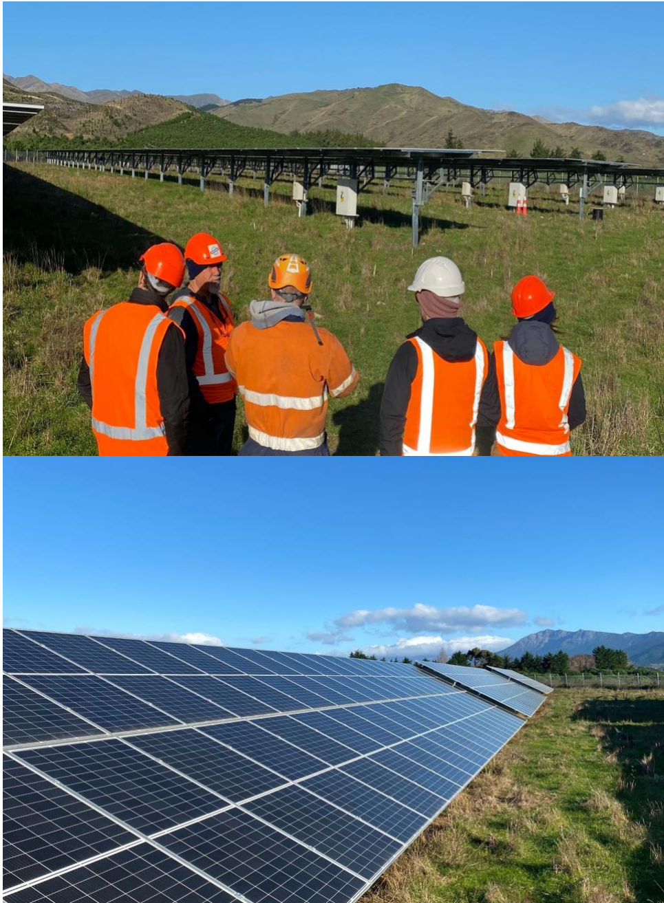
Figure 11: Photos from Site Visit to Wairau Valley Solar Farm June 2023
