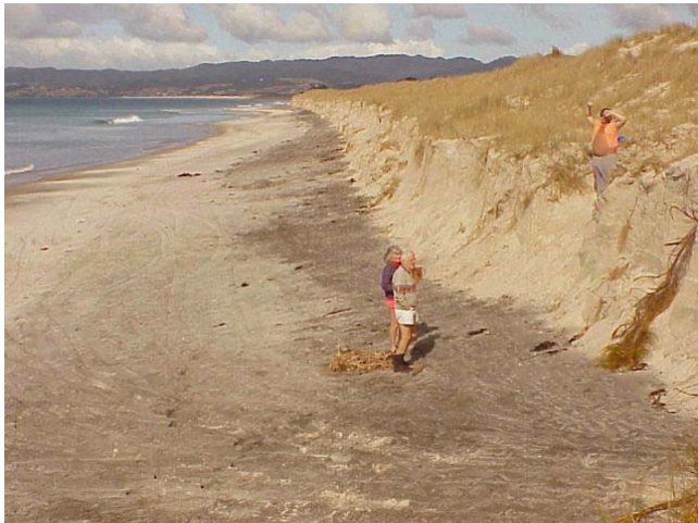
Foredune erosion at Bream Bay
