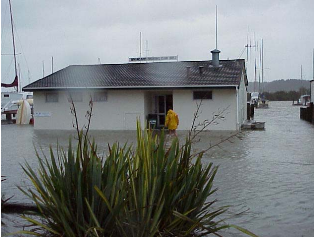
Flooding on the Hatea River, Whangarei
