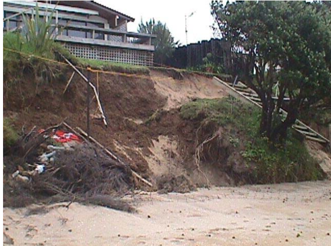
Erosion at Matapouri Bay
