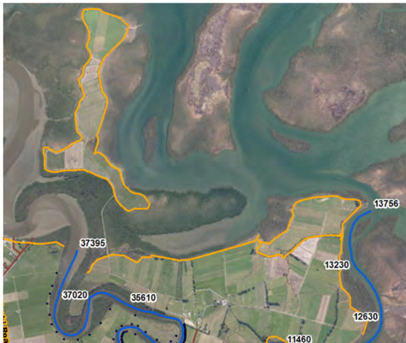
Figure 3-7: Dikes located at outfall of Whangatane Spillway and Awanui River
