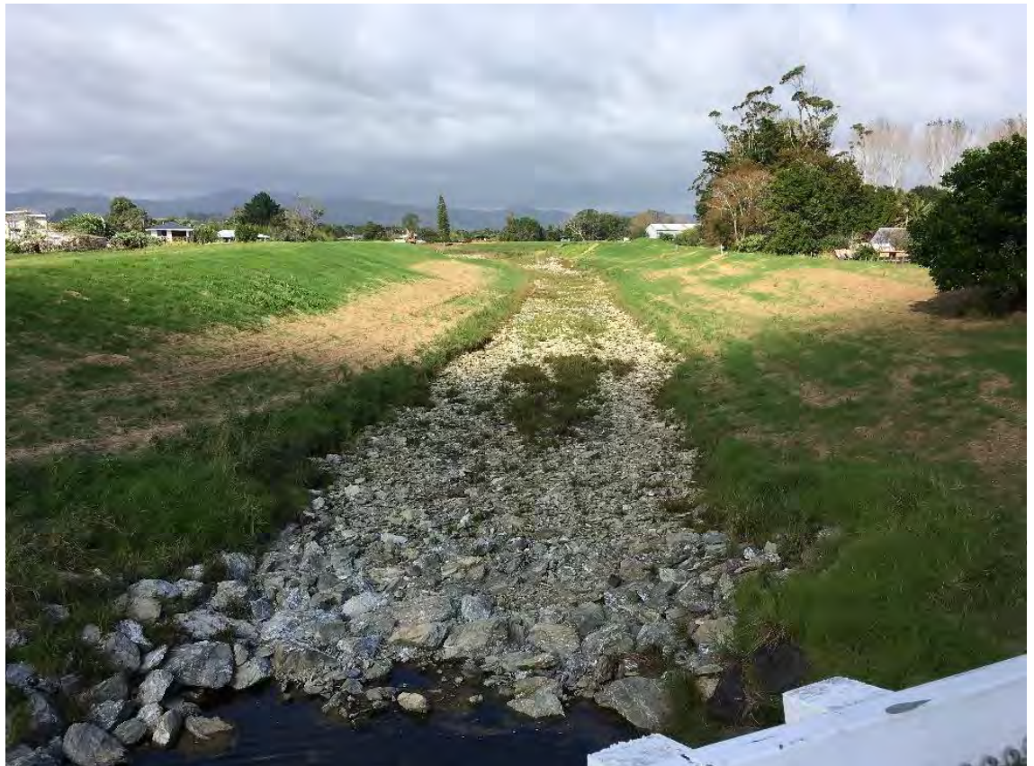
Figure 4-11 Whangatane Channel, upstream from Donald Rd 255m
