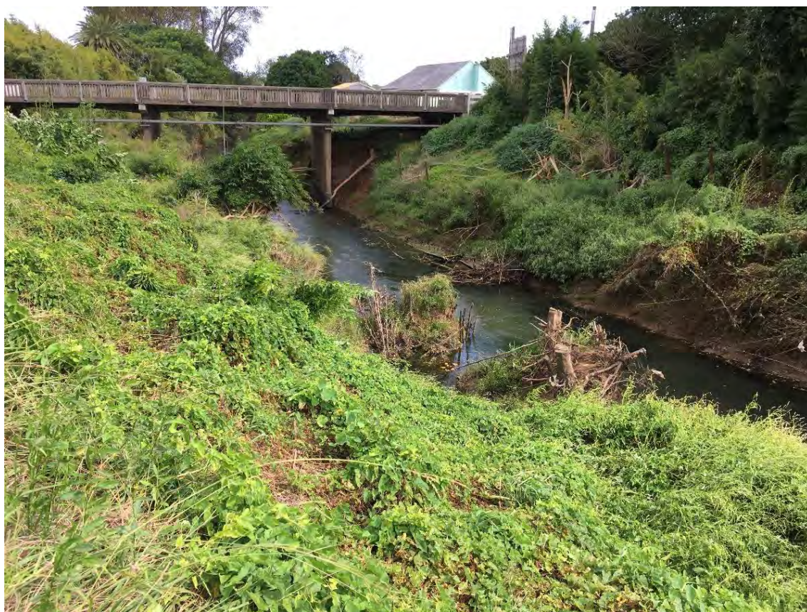
Figure 4-7 Awanui River: looking downstream to SH1 12368m
