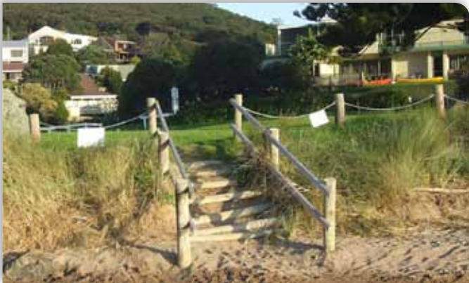
Walkways and fences can help plants establish and protect sensitive dune areas from trampling.
