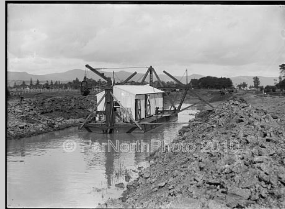
NC(370) Draining the Kaitaia Swamp Using Dredge
