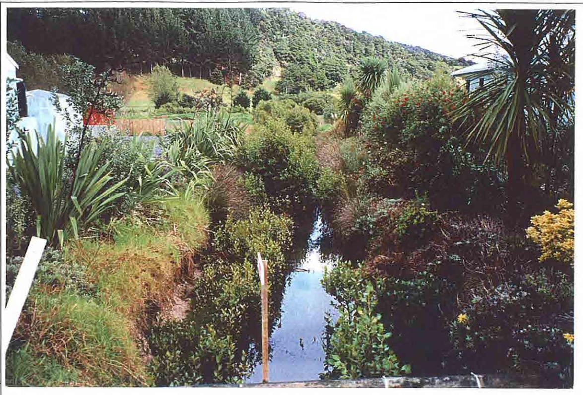
Photo 13: Tidal Drain under Waiotoi Rd - Downstream of PC15 – Looking South (note growth of mangroves in drain).
