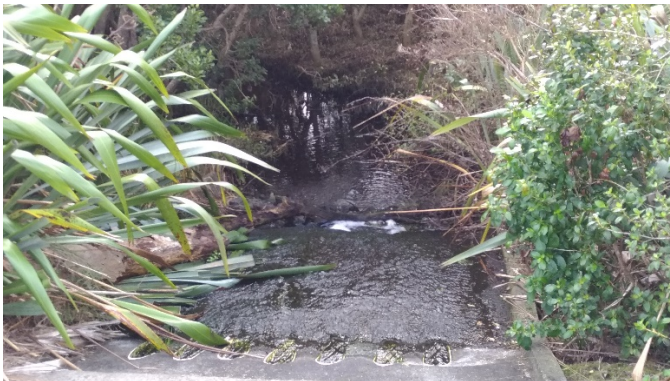
(b) Cascade discharge structure with treated wastewater flowing into Limeburners Creek
