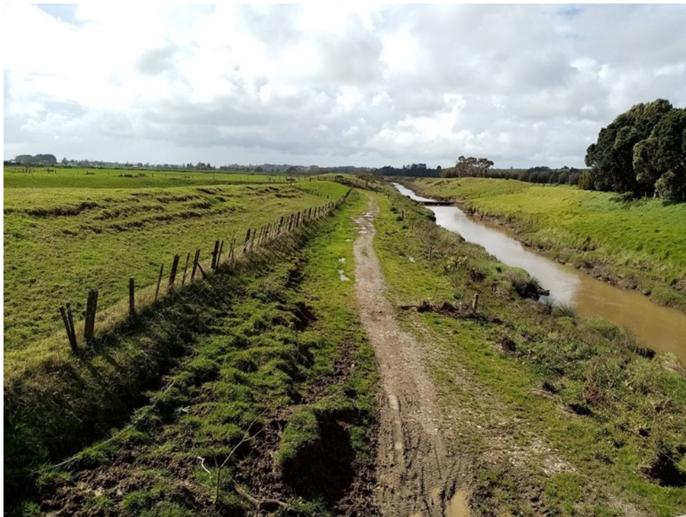
Figure 69: Looking north from Quarry Road at area of proposed benching area.
