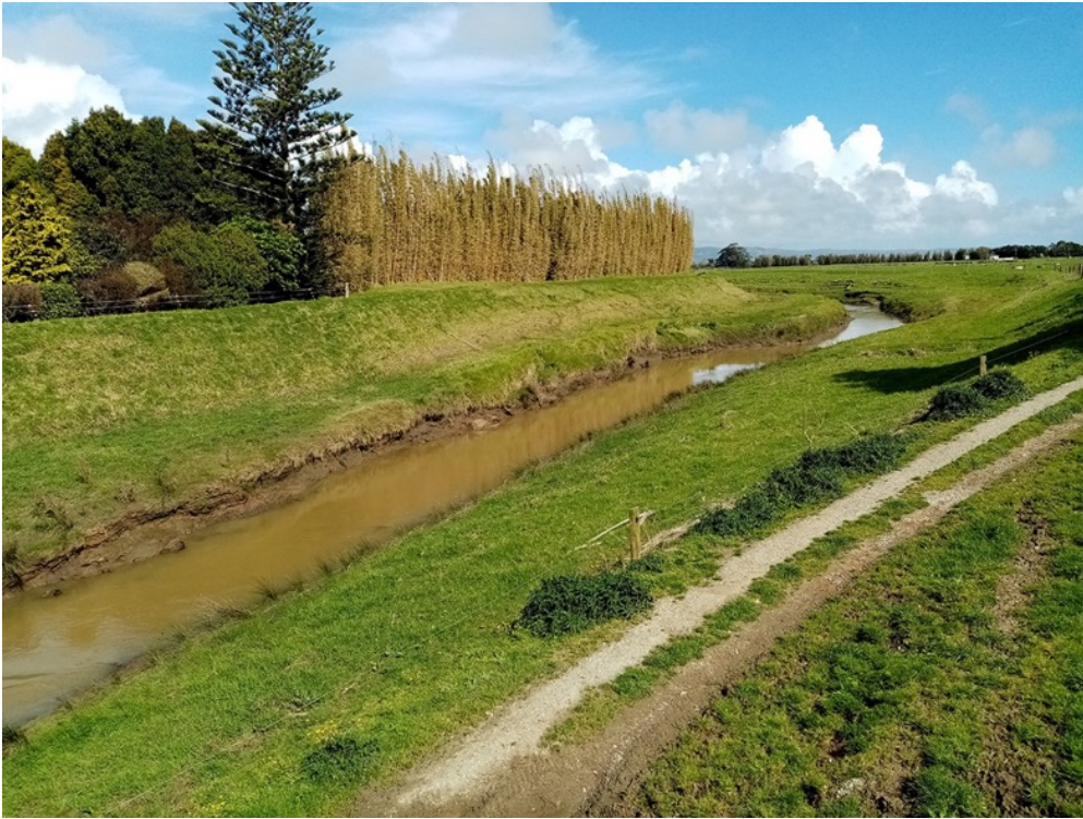
Figure 70: Looking south from Quarry Road at area to be benched on the left bank.
