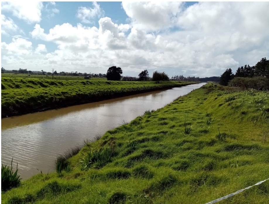
Looking north from SH10 at the Whangatane Spillway. Both banks will be benched and stopbanks upgraded.
