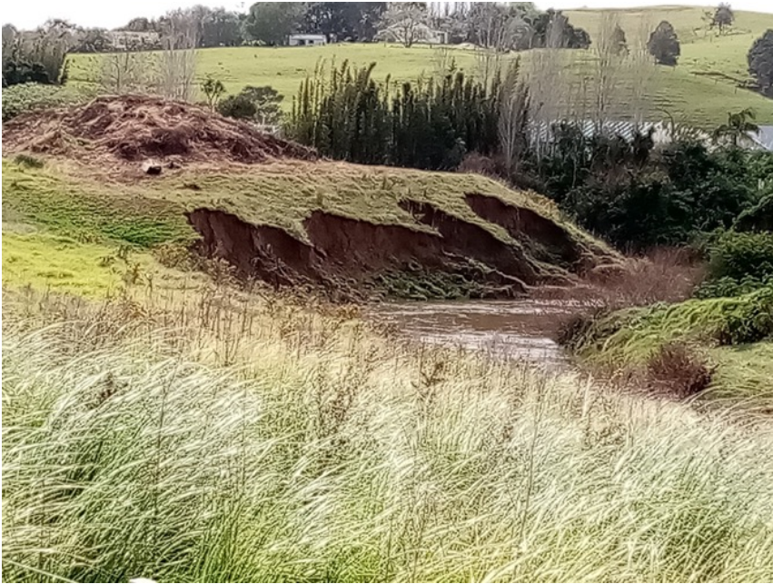
Figure 49: Eroding river bank and spoil mound on the east side of the Te Hiku Sports Hub.
