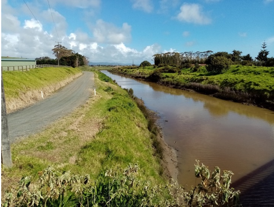
Figure 74: Looking south along the Whangatane Spillway from SH10. The right bank will be benched and the stopbank rebuilt.
