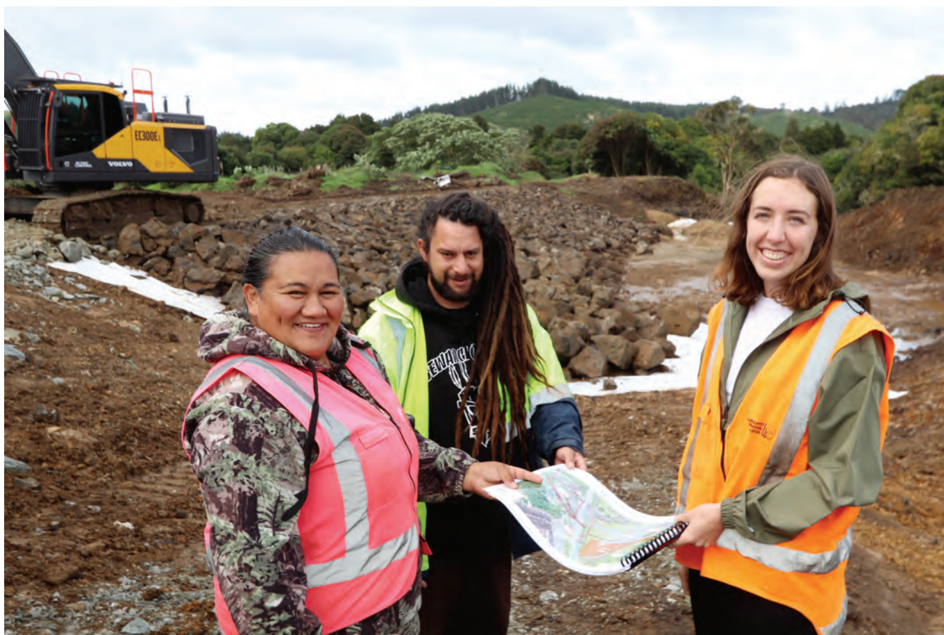
Stage One of the Otiria floodworks taking shape. From left, observers Pamela-Anne Ngohe-Simon and Danny Baker-Renata with Rivers Project Manager Meg Tyler.
