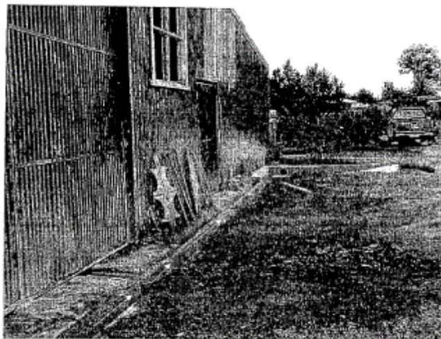
Wastewater from the precast building flows out into a drain and along into a settling pond. Arrows show direction of wastewater flow.
