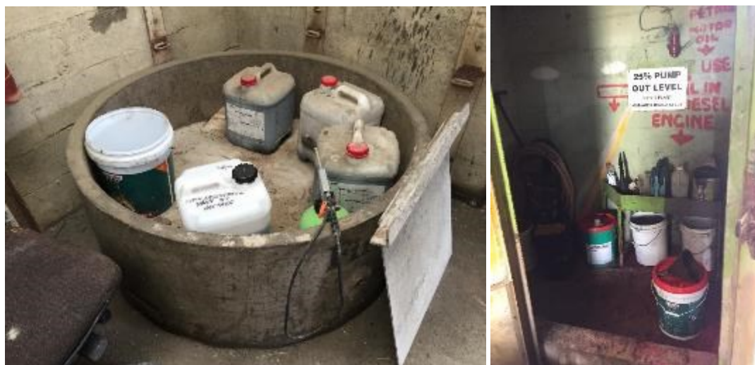
Photograph 17 & 18: Hydrocarbon/chemical bunding
