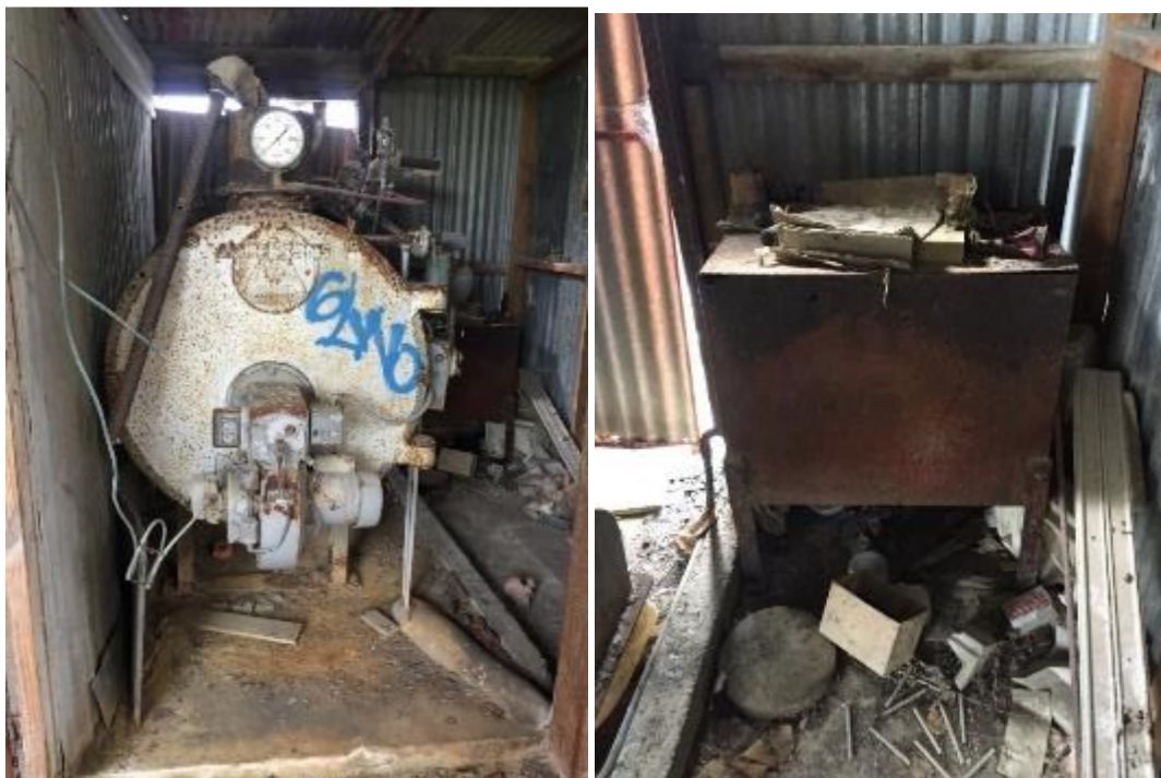
Photograph 11 & 12: Anderson Packaged Boiler and Day Tank in the Prestress Shed.
