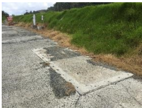
Photograph 33: Bund footprint of above ground storage tank(s)
