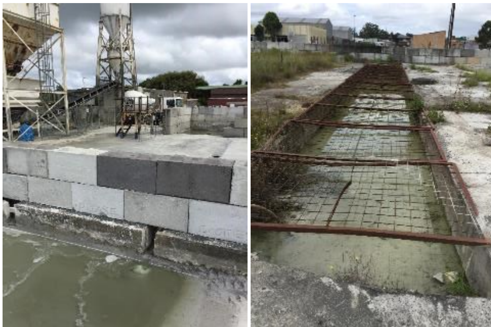
Photographs 25 & 26: Slurry pits/settlement ponds
