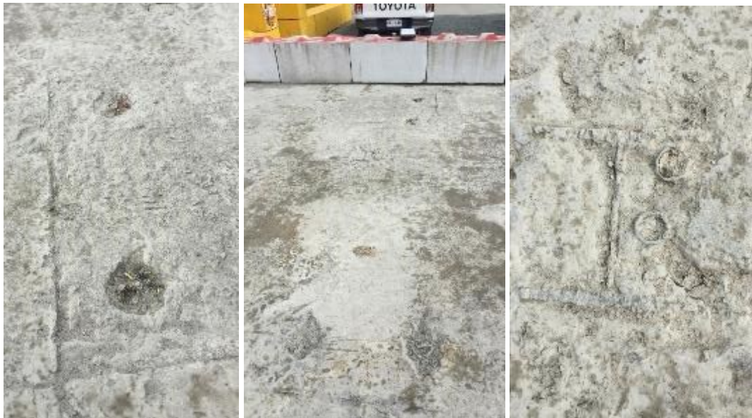
Photographs 34 - 36: Footings of fuel bowser and tank breather pipes
