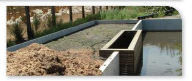
Weeping walls are designed to remove solids from farm dairy effluent. The removal of solids before irrigating means:
