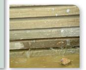
Sludge beds must be cleaned annually with the retained solids spread on pasture or crop paddocks. The weeping walls should be pressure washed while the sludge beds are empty. Any broken slats or knot holes can be repaired using plywood strips.
