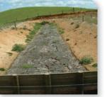
the concrete apron under the weeping wall must be slightly lower than the bottom of the sludge bed.
