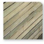
Correct design and installation is critical if a weeping wall is to work effectively. The required wall area is typically one square metre for every 100 cows but with a minimum of five square metres for each wall. The recommended gap between slats for effluent from the dairy is eight to 10mm and for feed pads 15 to 18mm.
