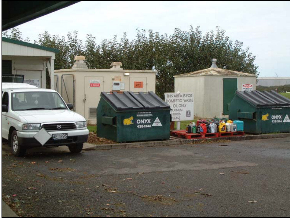
Hazardous waste store at Pohe Island
