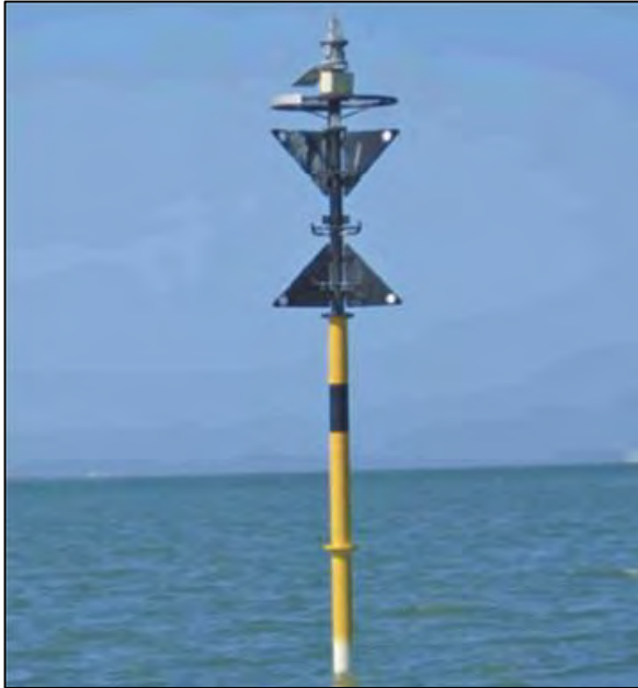
Figure 1.5.15.1: Example of proposed West Cardinal Beacon
