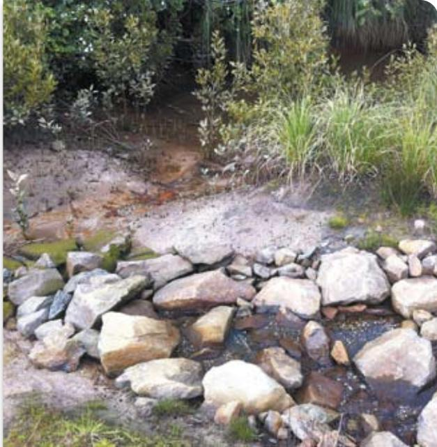
A rock ramp fish pass, with rocks forming a zigzag pattern across the stream bed to reduce flow and provide pockets of still water/eddies where fish can rest as they move upstream.
