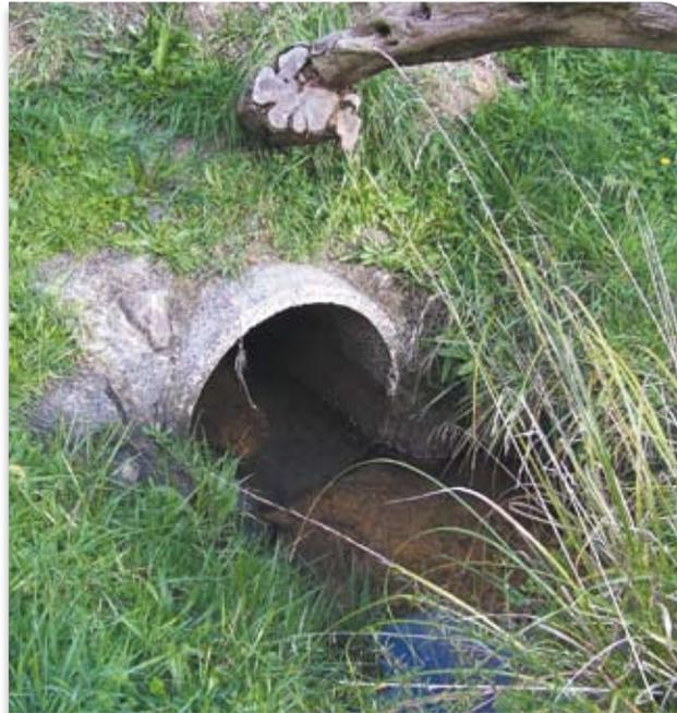
A well-designed culvert allows for fish to move through as part of their lifecycle
