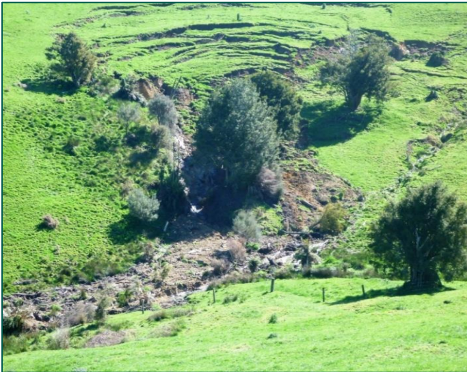
Shallow earthflow triggered by stream undermining the toe of the slope and continual saturation from a spring.
