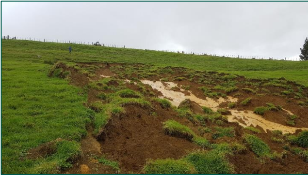
Shallow slip caused by intense rainfall infiltrating down through cracks formed in summer lubricating the layer between the topsoil and harder subsoil creating a slip plane (i.e., a greasy back)
