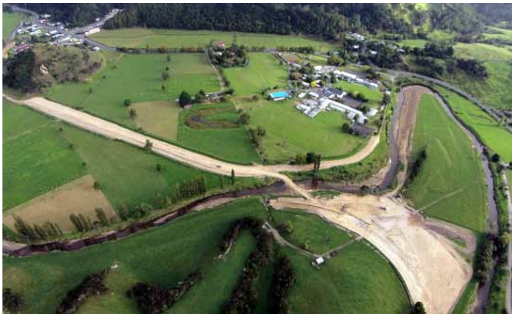
Major works to reduce flood impacts in Kaeo were completed
