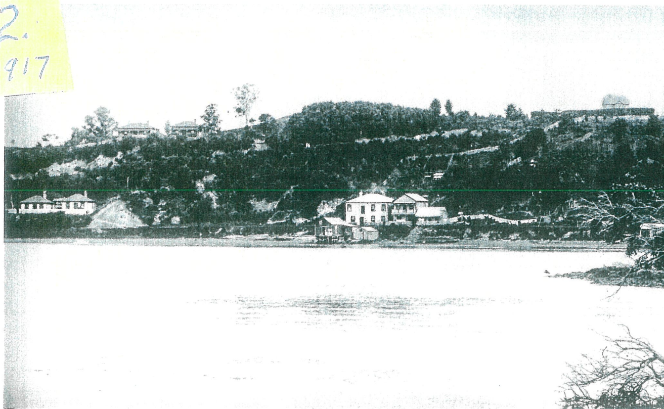
2. 1917. Opua main beach. Two railway houses, boarding-house, Allens Bakery, store on Beechey Street. Goods shed on foreshore.
