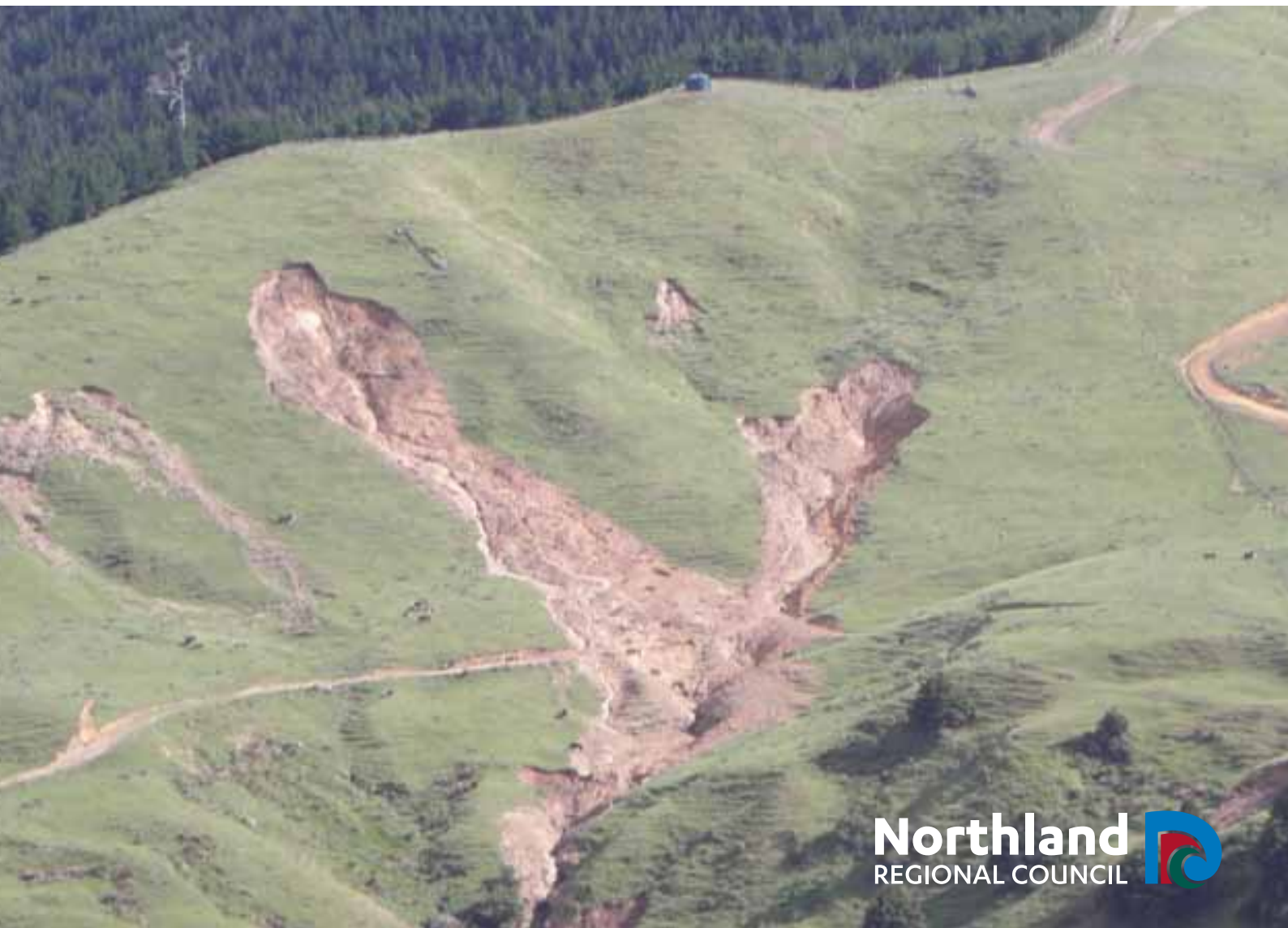
Slipping on Waimatenui hill soil (YNH)
