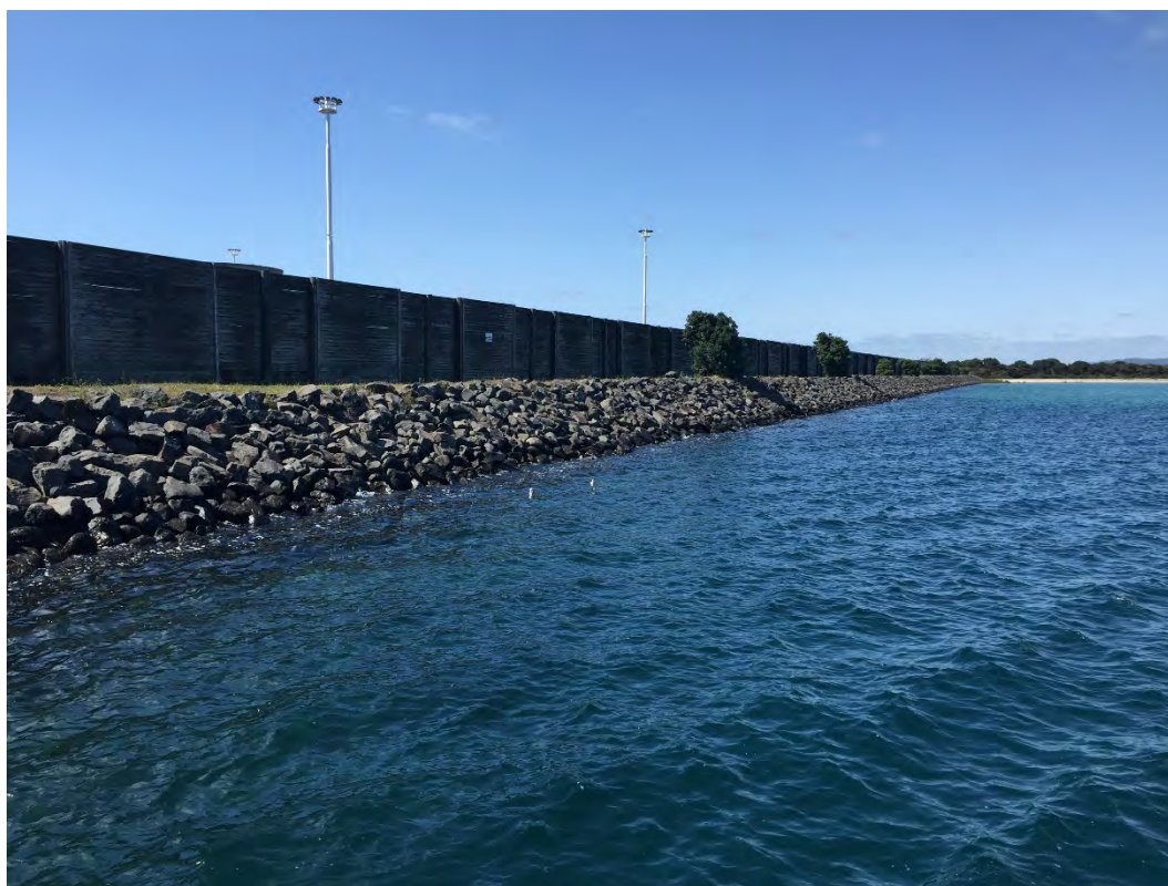
Photo 8: Riprap revetment along Northport western boundary
