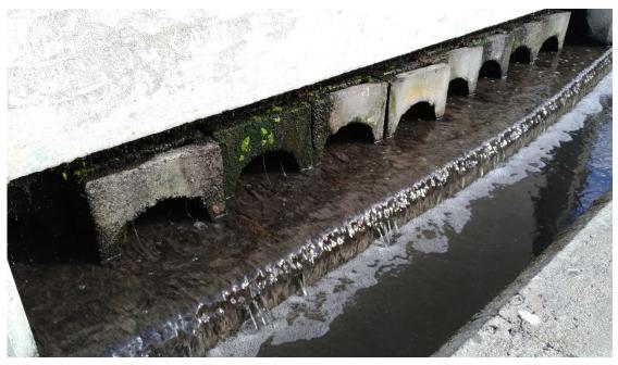
Figure 7 - Trickling Filters – outlet launder
