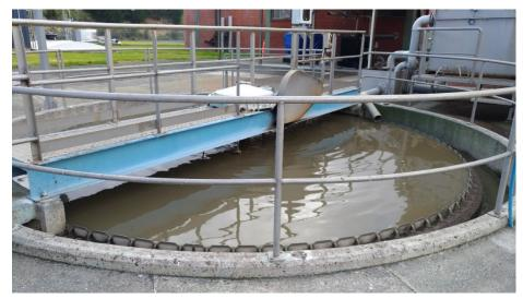
Figure 16 - Primary sludge gravity thickener
