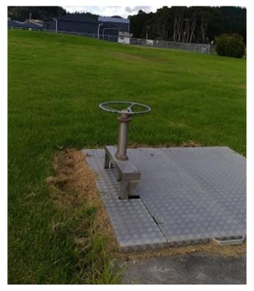
Figure 15 - Emergency outfall isolation valve (with manual padlock)
