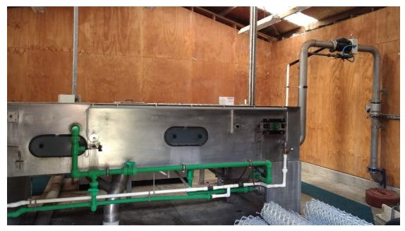
Figure 17 - WAS gravity belt thickener
