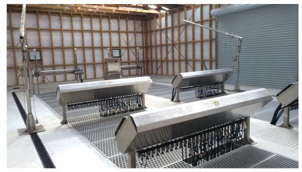
Figure 13 – High Flow UV treatment facility
