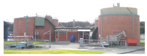
Figure 18 - Digester Tanks and Gravity Thickeners (buried foreground)
