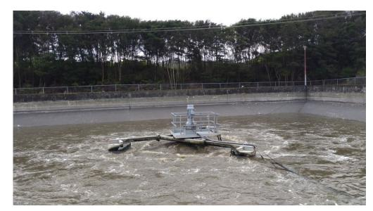
Figure 5 - Equalisation Basin and surface aerator
