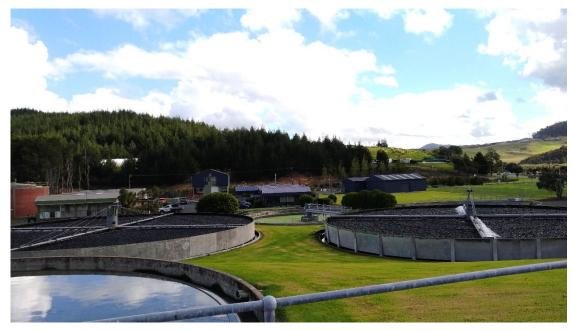
Figure 6 - Trickling Filters
