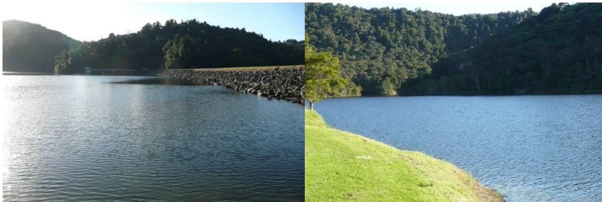
The Whau Dam (left) and looking away from the dam (right).
