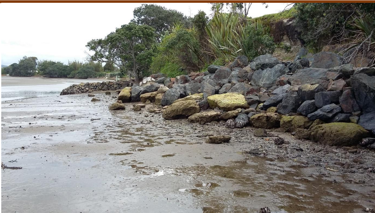
Photo 10: Series of existing hard shore protection structures, small jetties and access ways located approximately 100 to 500 metres southwest of proposed wharf
