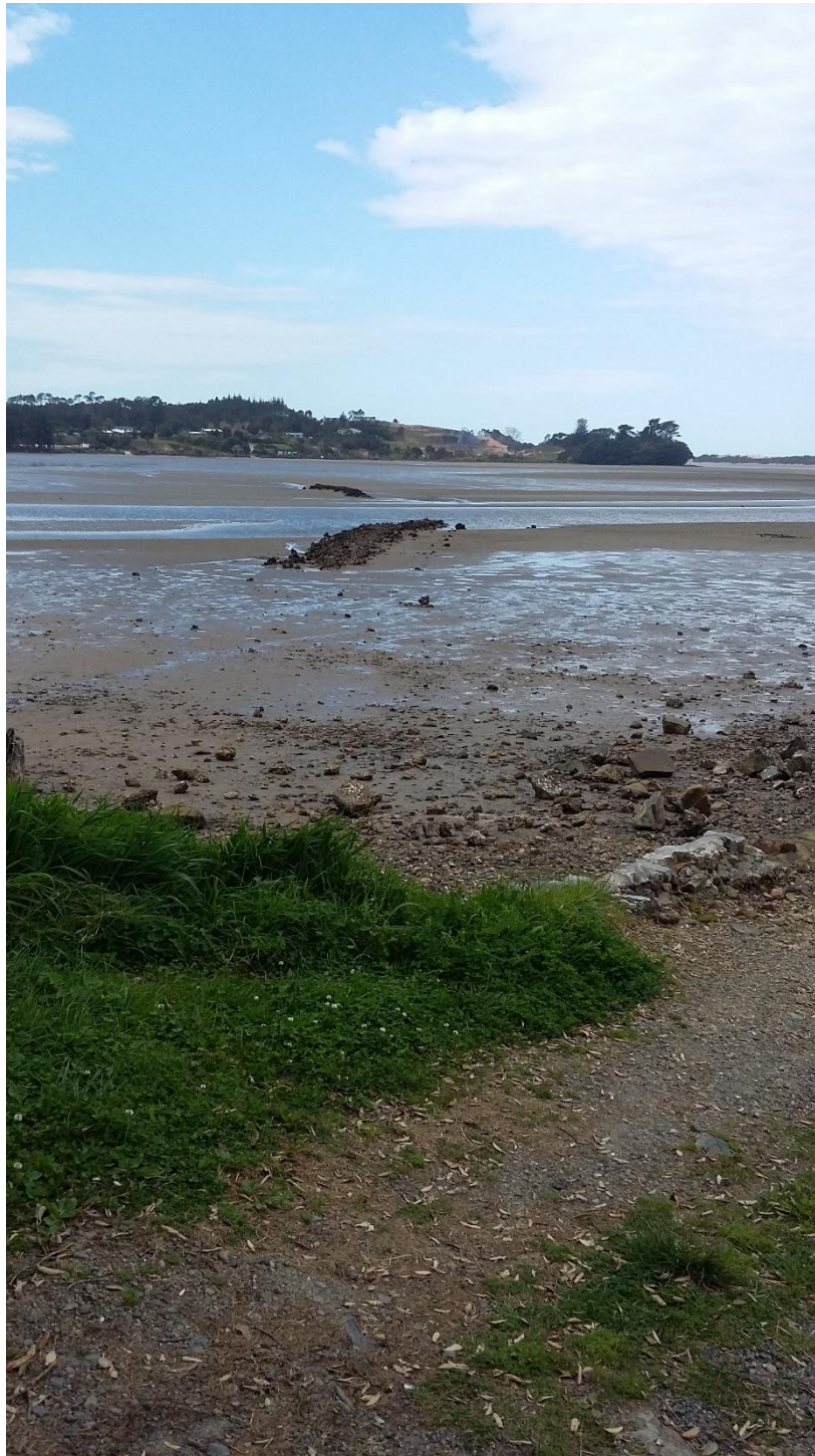
Photo 2: Historic channel training groynes & remnant cut-off piles
