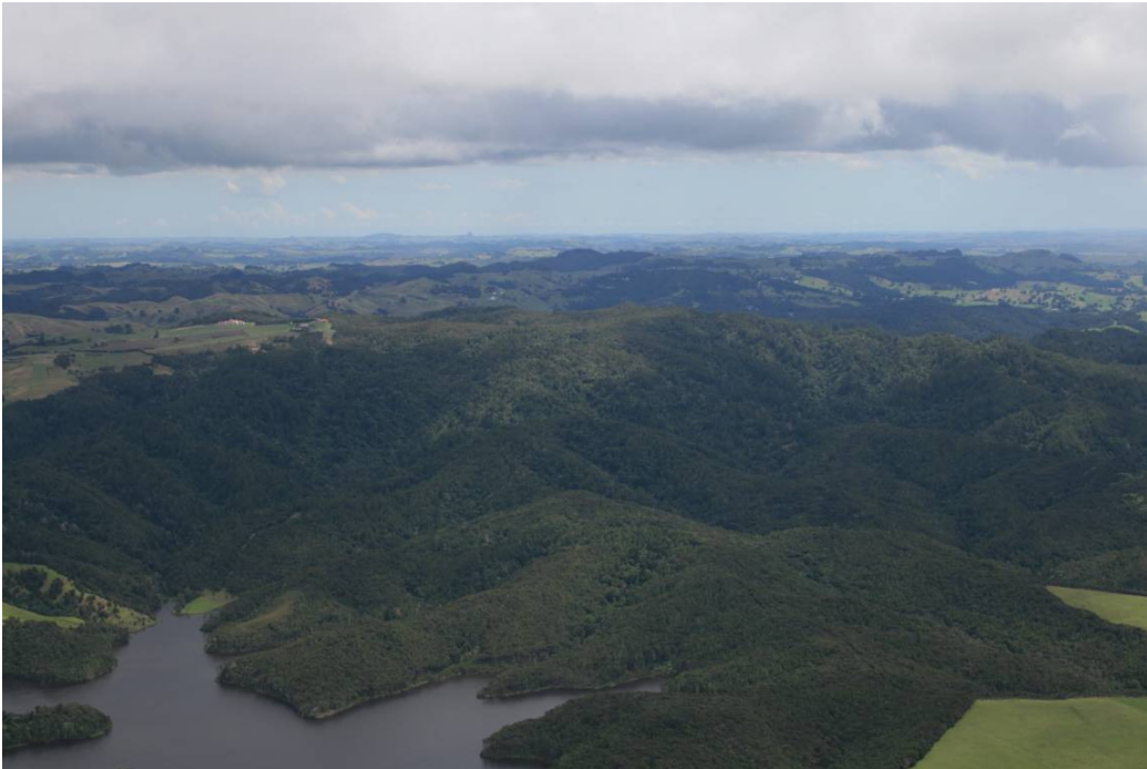
Ruakaka Forest and Wilsons Dam from east
