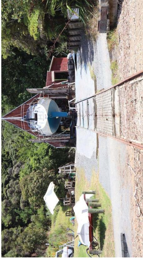
**Photograph 6:** A view up the slipway as it currently stands, with the existing containment drain positioned roughly half way up the rails and the perforated walkway crossing immediately below that. The small taper of wall to left marks the apex of a concrete dinghy ramp. Timber to lower right is the landing of the existing wharf.
