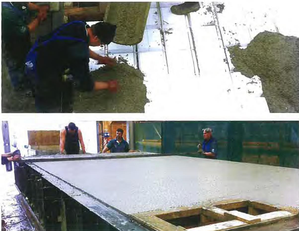
Figure 8: Concrete pontoon casting process.
