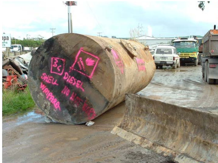
Photo: De-commissioned diesel tank
