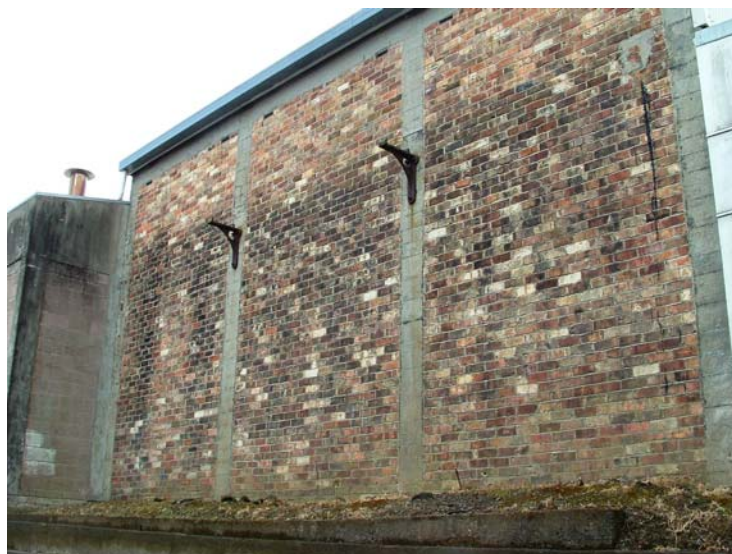
Photo: Exterior of former Gasworks in Whangarei
