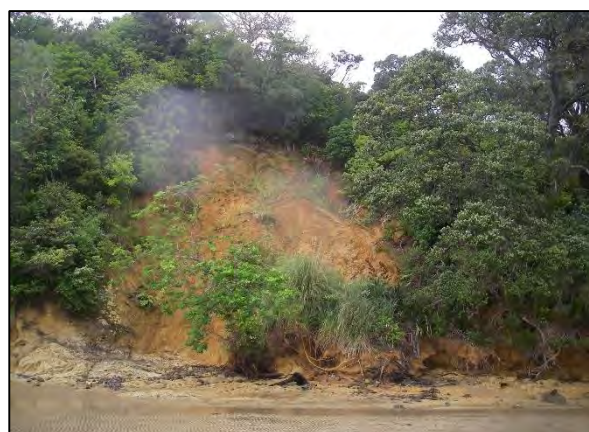
Site Photograph C (southern end - cliff)
