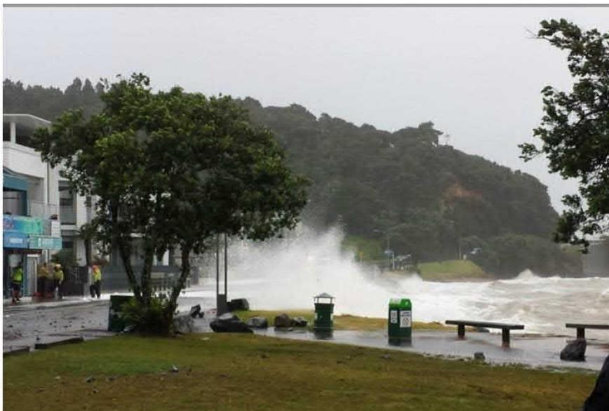
Figure 4-4: Overtopping of the rock revetment along the Paihia CBD foreshore during a storm event in 2014 (source: R Griffin)
