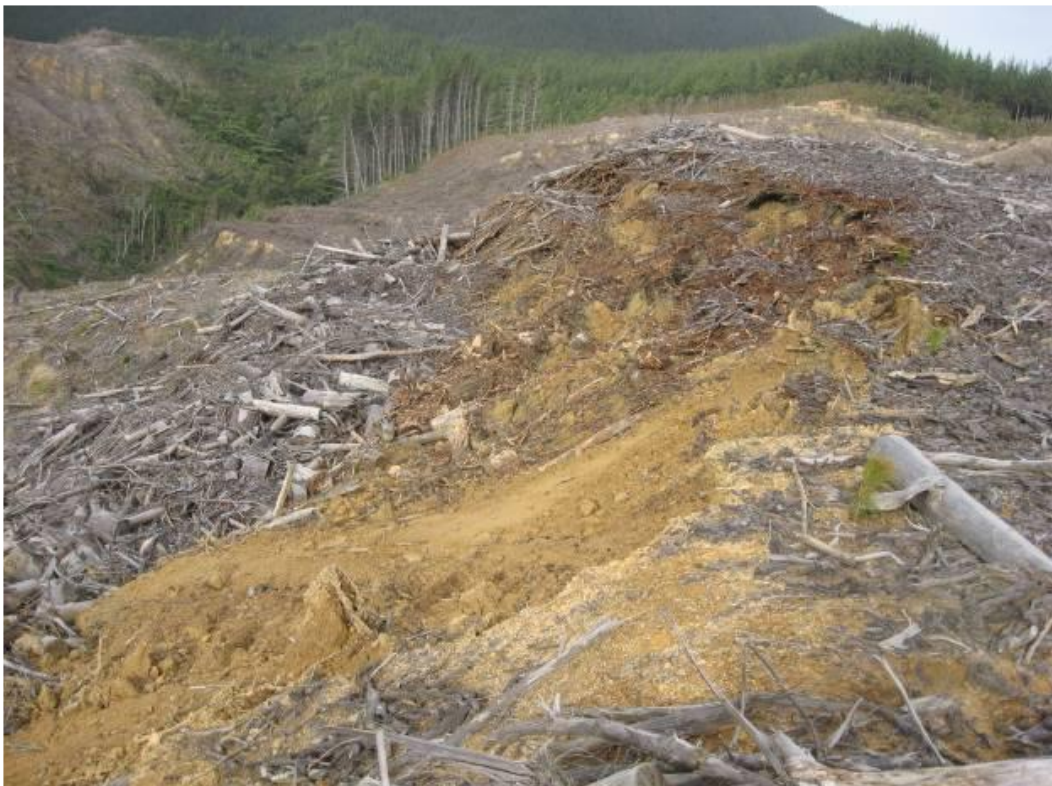
A slumped landing as a result of slash left on fill areas combined with poor water control.
