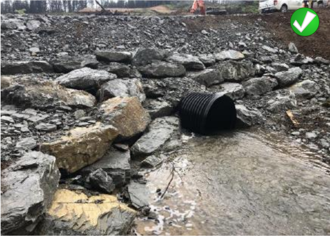
Compliant fish passage structure
