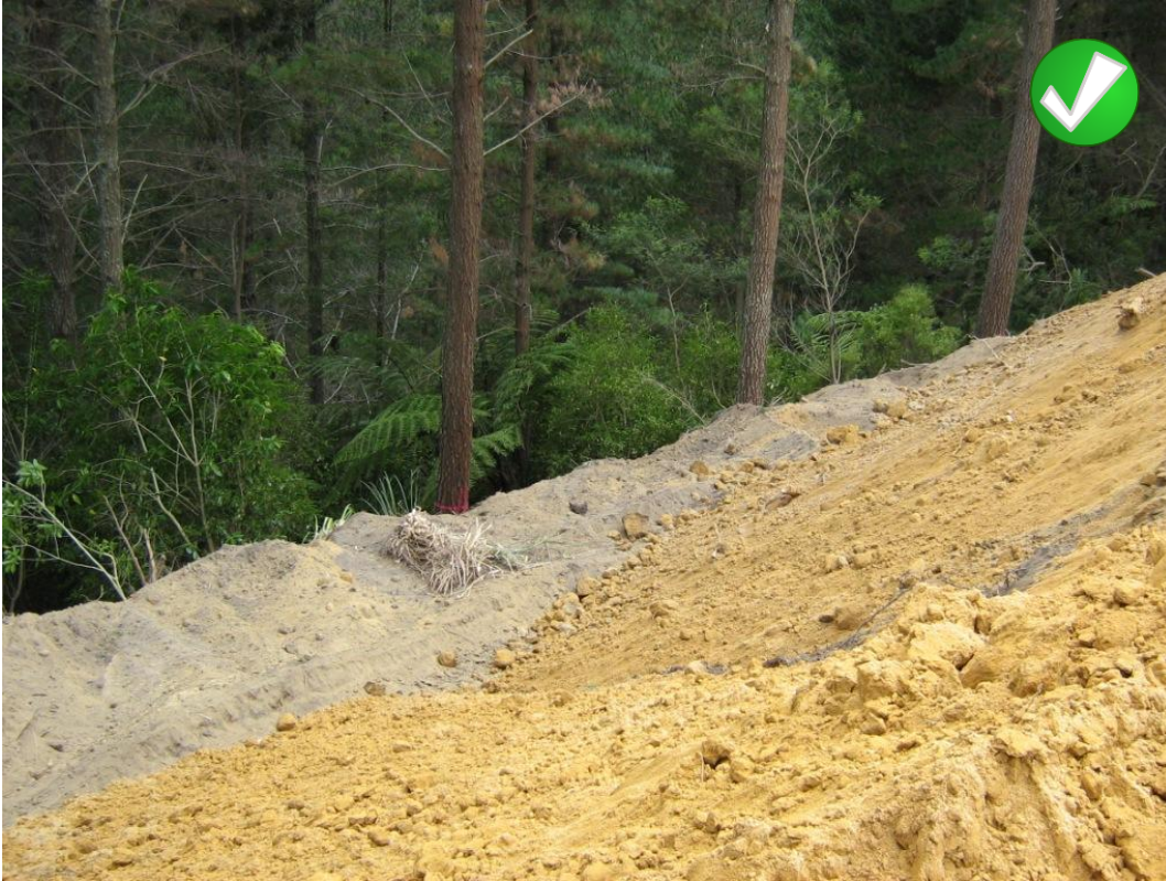
A visible bench with stumps and slash stored in stable location.
