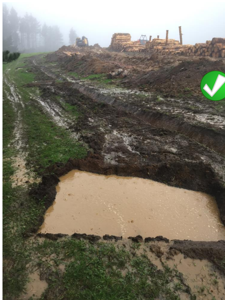
A landing with effective water diversions and well-spaced sediment traps to service the area.
