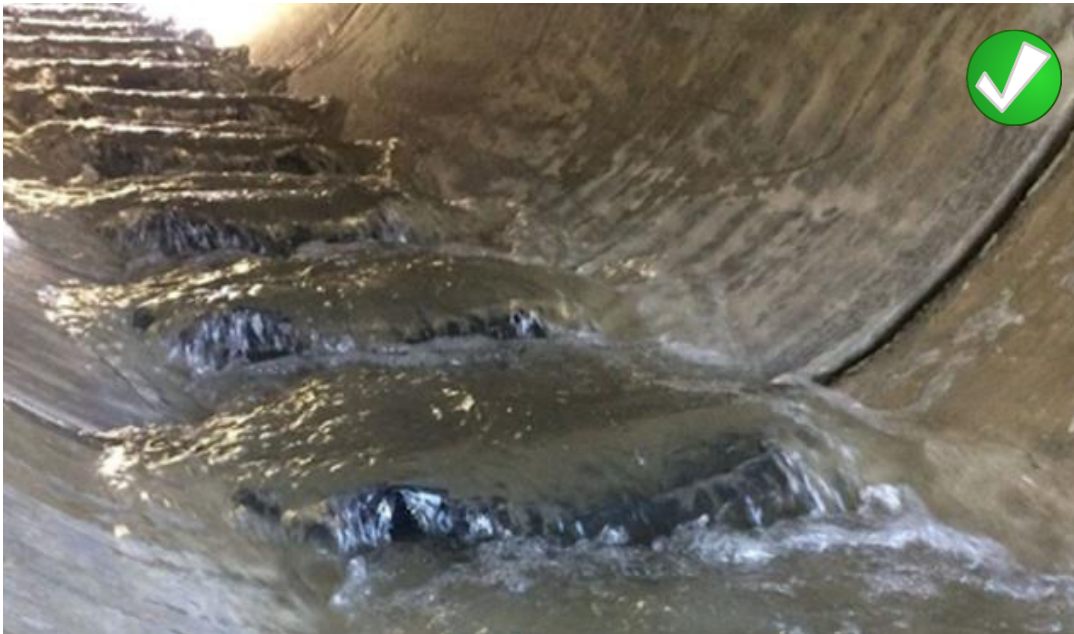
Compliant fish passage structure
