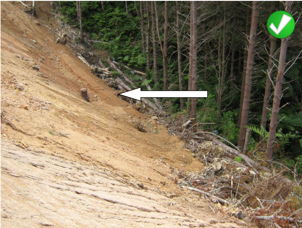
A visible bench with stumps and slash stored in stable location.
