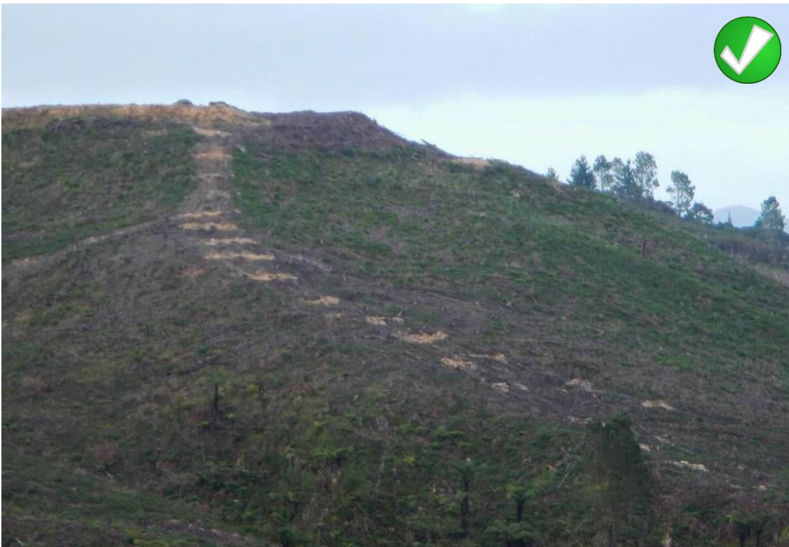
Photo below shows correct use of cut-outs for water control
