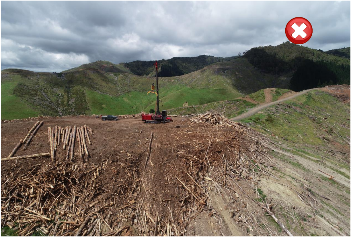
A slumped landing as a result of slash left on fill areas combined with poor water control.
